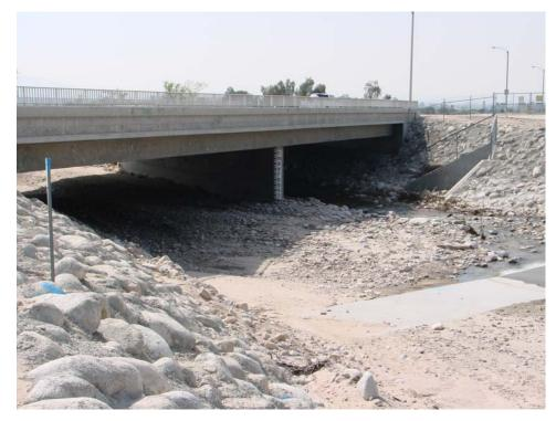
The Plunge Creek Bridge had to be replaced A hydrology and hydraulics study was also and the Plunge Creek Channel had to be improved per San Bernardino County Flood Control (SBCFC) requirements. JBA was retained to perform a scour analysis to determine the proper depth of bridge abutments and to engineer necessary slope protection for Plunge Creek.
