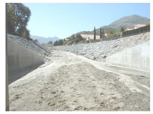
A hydrology study was prepared in relation to a large subdivision development in Reche Canyon. The Reche Canyon Channel ran through the property and needed to be improved. The property in the area in of the channel was in a floodplain as designated by FEMA which required the filing of a study with the Corps of Engineers to remove the area from FEMA's jurisdiction. A channel had to be constructed with appropriate inlet/outlet structures and a bridge.
